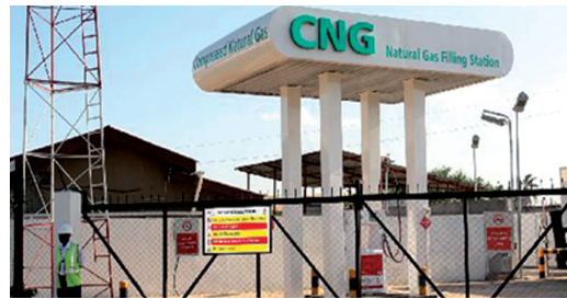
Figure 8: CNG Filling Station in Dar es Salaam - Ubungo
